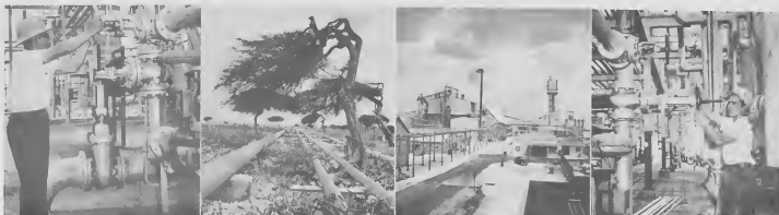
THE OPENING of a valve, the starting of a pump..... these basic operations will send HARRIMENTO di un valvola, startamento di un pomp..... e trabasnan basico aki te manda Lago's fuel gas through ten miles of pipeline to ACI where it is used as feed gas for ammonia production. Lago su fuel gas door di diez milla di tubo pa ACI na unda e gas ta ser usá pa produccion di amoníaco.
